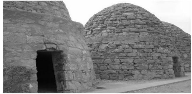
excavation. The clay was poured into brick molds, set to dry, and then removed from the molds. An igloo-shaped kiln of the dried bricks was created and then the dried bricks were fired. Wood would be placed into the kiln. The harder glazed bricks would be nearest the heat source while the softer bricks were further from the scorching temperatures. Both the exterior and interior walls are 19” thick. The Jarrot Mansion brochure states,
