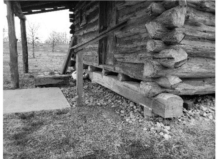
With these new logs and flashing, the rest of the cabin should stay in great shape for a long time. We will be stabilizing the north side of the cabin and repairing both sets of steps this winter and spring as weather permits. Thanks to the Lewis & Clark National Historic Trail for the assistance in seeing this work completed.
